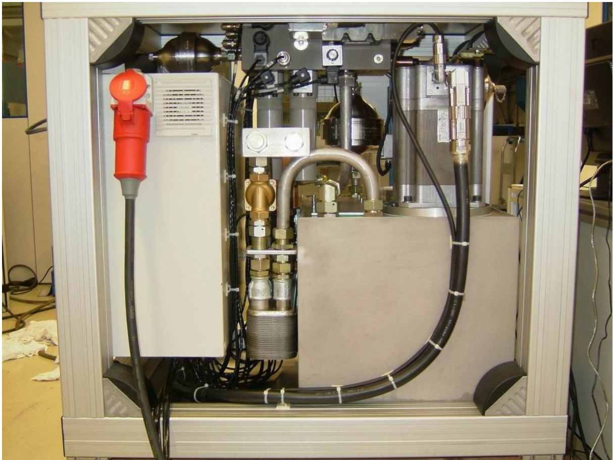
The hardware is a compact design, but all elements are still easily accessible.
